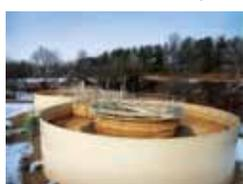
This 740,000-gpd system almost exclusively treats domestic wastewater. The former system was a field-erected activated sludge plant rated for 275,000 gpd.
