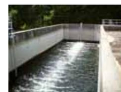
This 1.2-mgd system also almost exclusively treats domestic wastewater. The former system was dual-basin constant-flow SBR activated sludge plant rated
