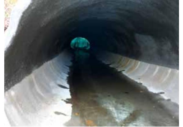
**Left: Culverts made of bolted corrugated metal plates sometimes fail at seams and boltholes. Middle: An example of a culvert with a paved invert and uncompromised upper portions. Right: A completely rehabilitated arched metal culvert; the upper arch was spraycasted with cementitious grout.**
