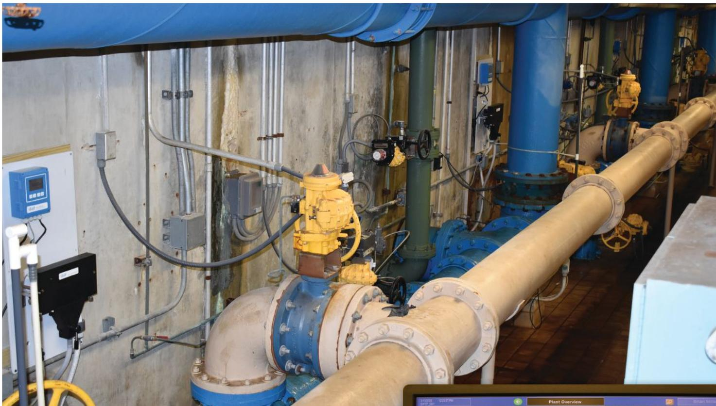
Top: Non-contact turbidimeters reduced the maintenance burden for Greer CPW.
