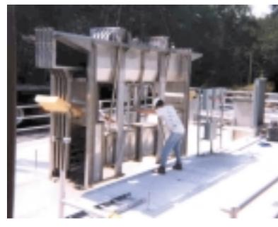
**Figure 2: Downstream Serpentine Weir in Channel**
