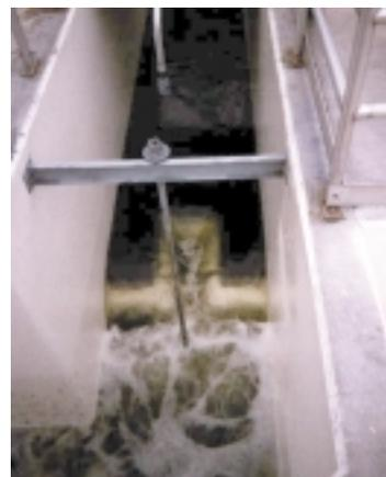
**Figure 3: Flow Control Gate in Closed Position**
