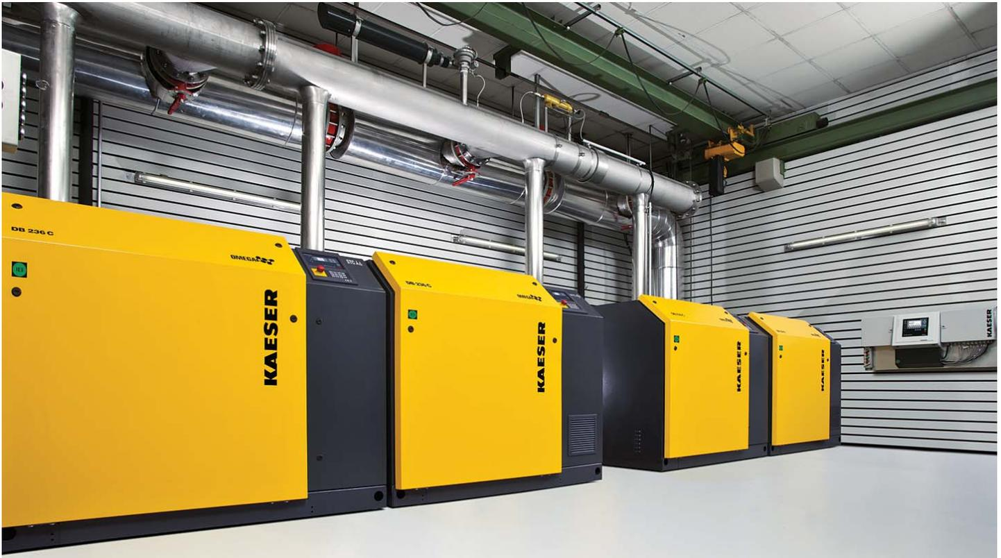
**FIGURE 4:** Multiple, integrated blower packages controlled with a system master controller offer an energy-efficient and reliable solution for wastewater treatment plants.
