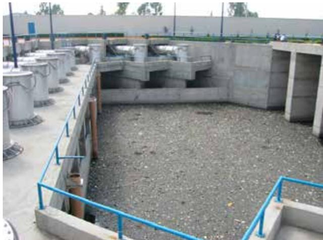
Figure 1: A wastewater sump covered with floating debris.
